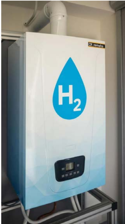
Figure 9: Hydrogen boiler, capable of using 100% hydrogen as fuel (Baxi Heating)
