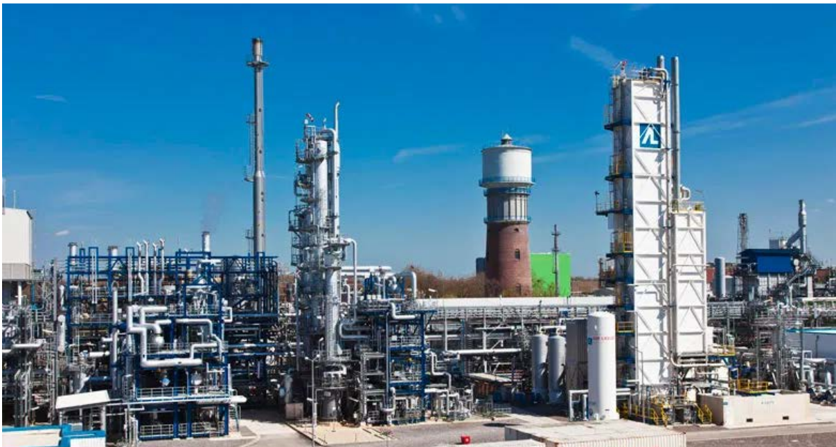
Figure 5: Steam methane reforming plant in Dormagen, Germany
