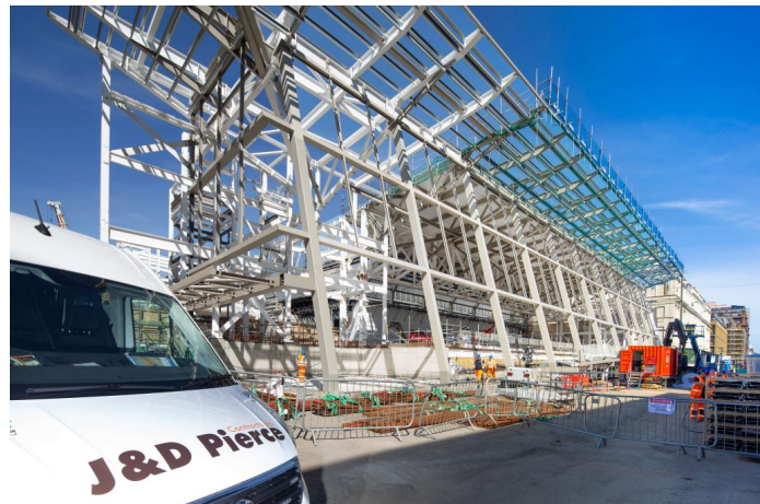
New Glasgow Queen Street Station in Construction
